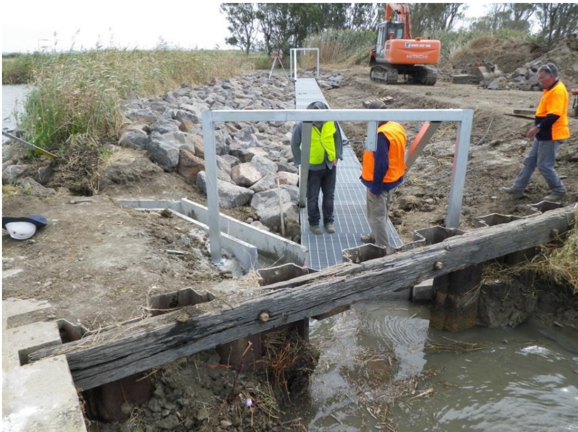
A trench is dug for the attraction flow channel. Concrete is poured around the culvert units and attraction flow channel to secure the structure. Rock is placed along the banks of the fishway to reinforce the banks against erosion, gantry for gates installed and remaining concrete poured.
