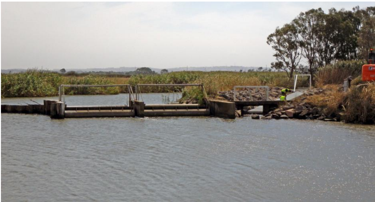
Entrance placed to right of main gates of weir. A small rock groin places fishway flow adjacent to the abutment wall.
