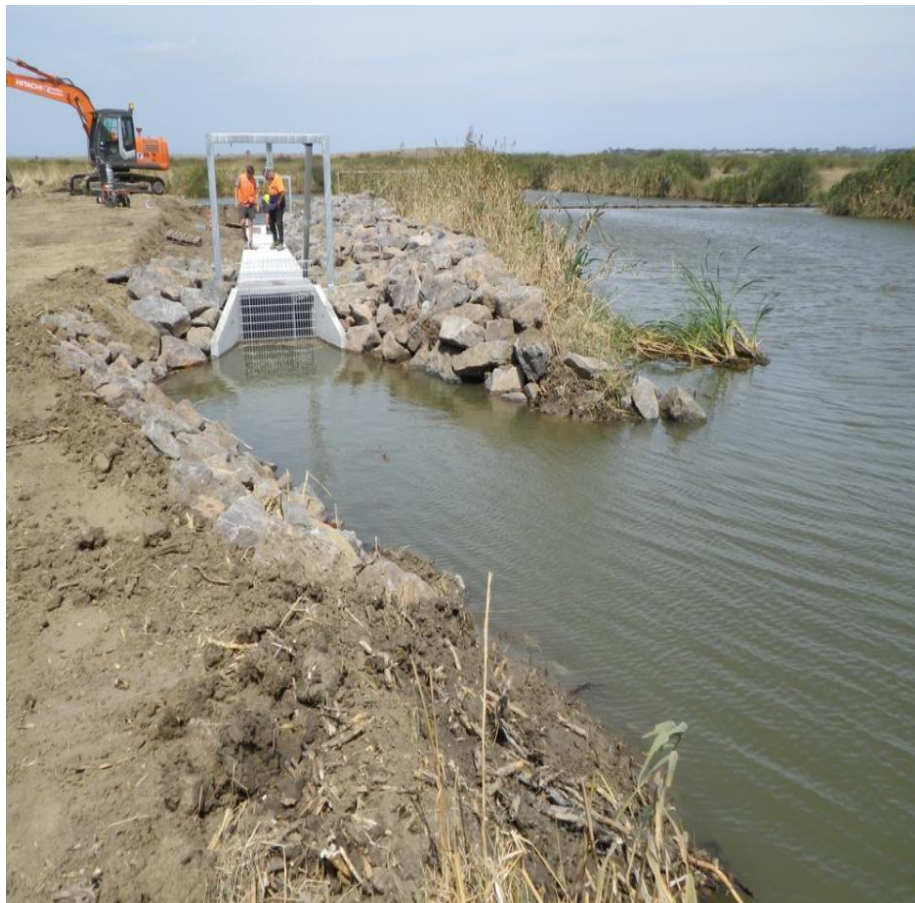
Upstream exit recessed into bank and rock lined (temporary grate in place).
