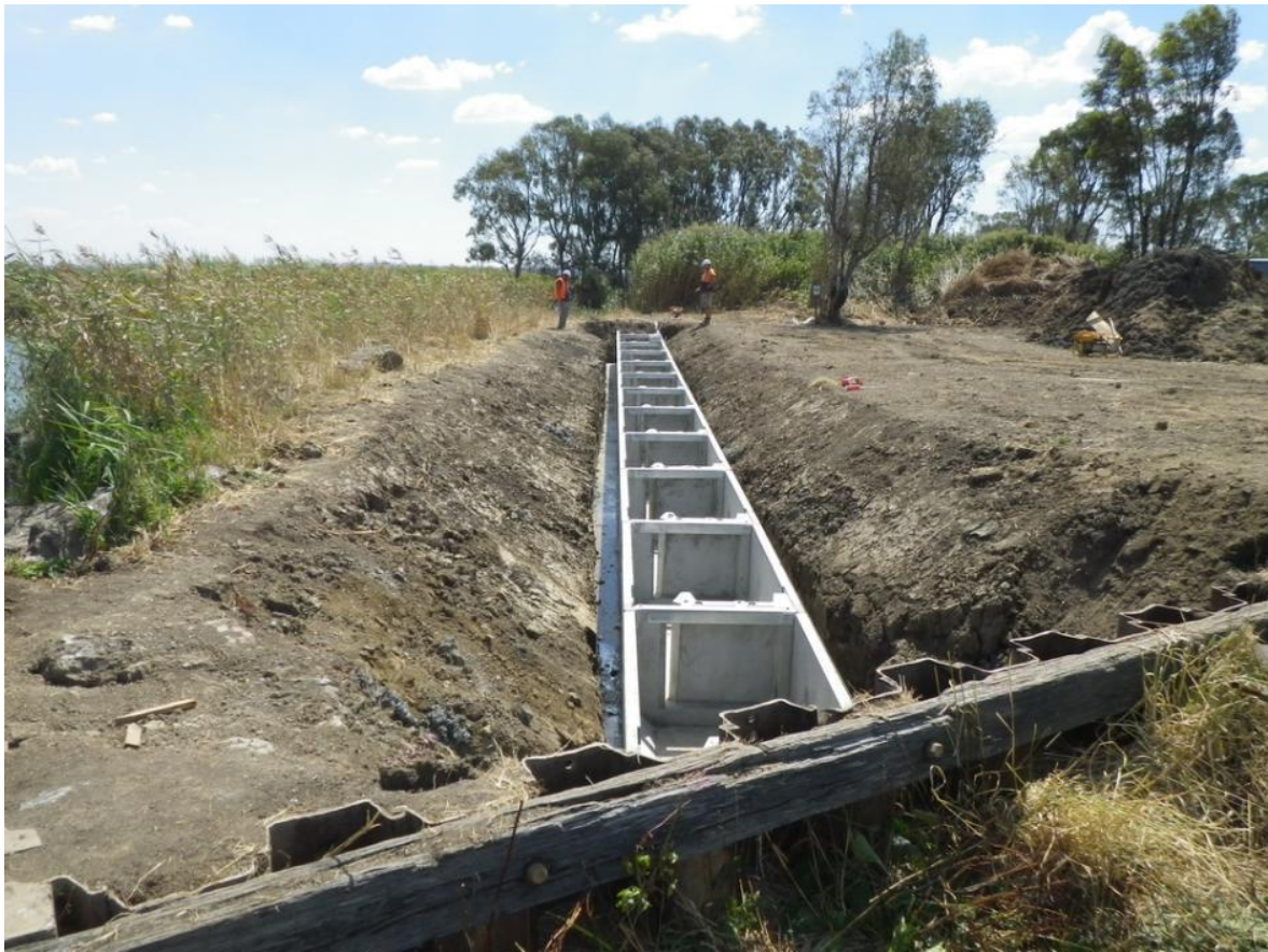
Upside down culvert units are placed on the slab which form the fishway channel.
