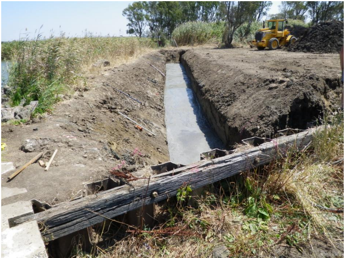
Channel is completed and a blinding concrete base is poured to help slab construction.
