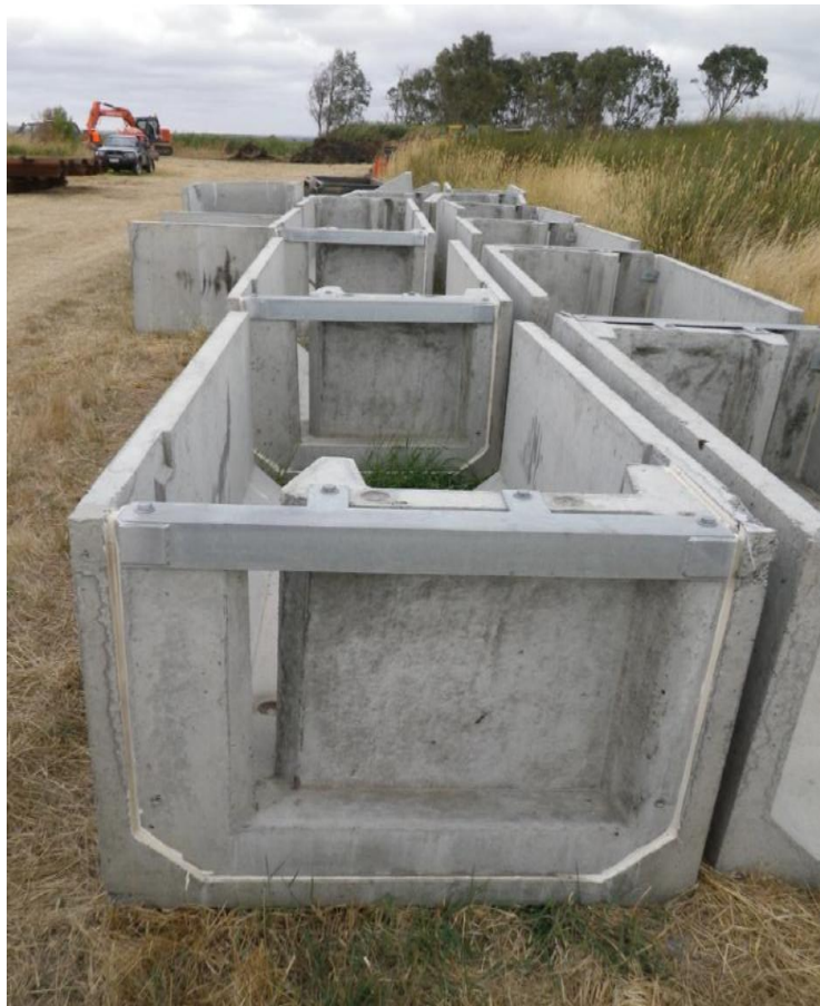
Culvert units used in the fishway construction.
