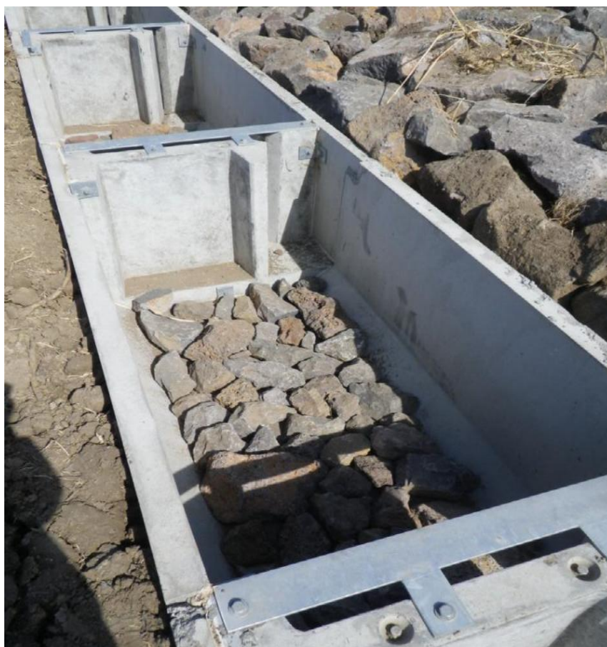
Rocks were placed in the bottom of the fishway to enhance roughening.
