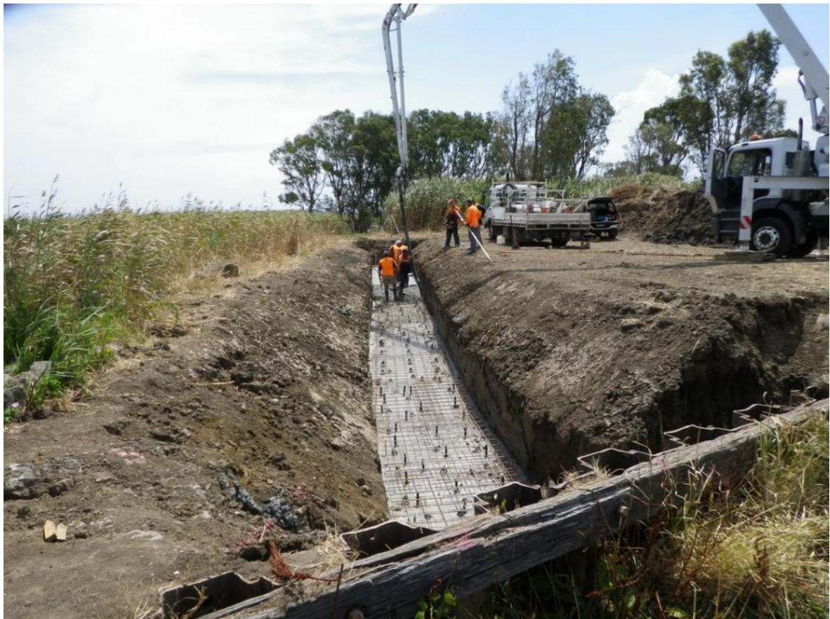
The following day some water enters the site and is pumped and slab formed and poured.
