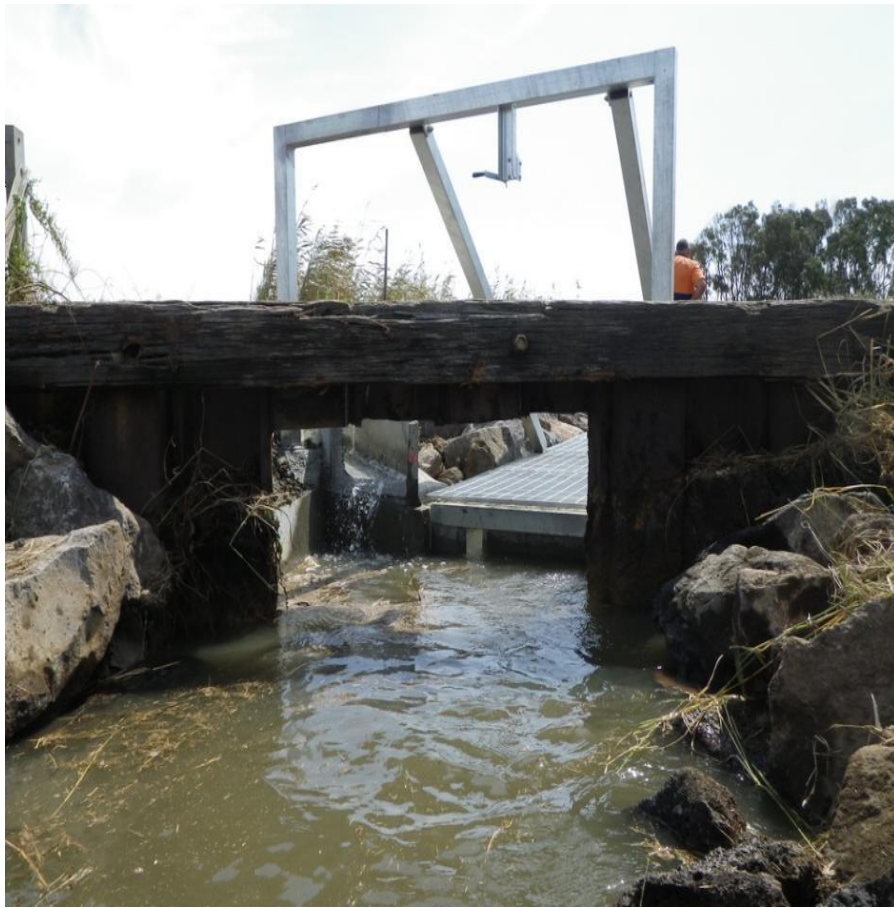
Entrance set behind sheet pile wall to reduce construction time and maximise site safety and retain weir integrity (hence a hole rather than a slot).
