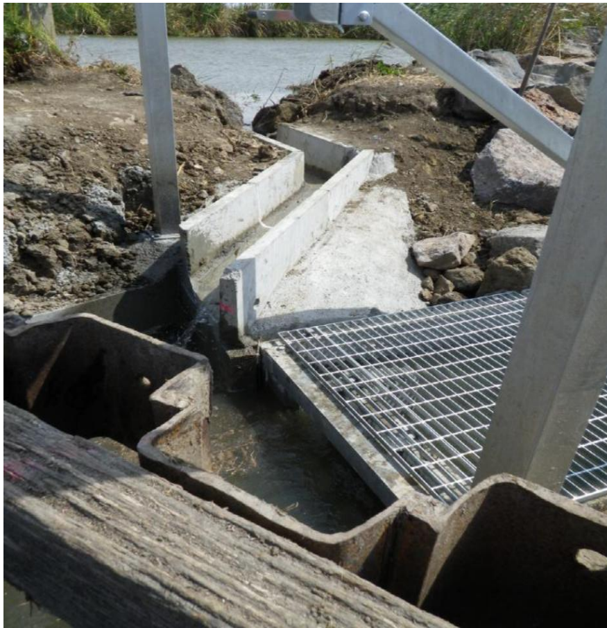
An attraction flow channel provides extra water to fishway entrance. Plunging flow chosen to maximise noise attraction. Attraction flow operates to 100mm below FSL (maximum allowed)
