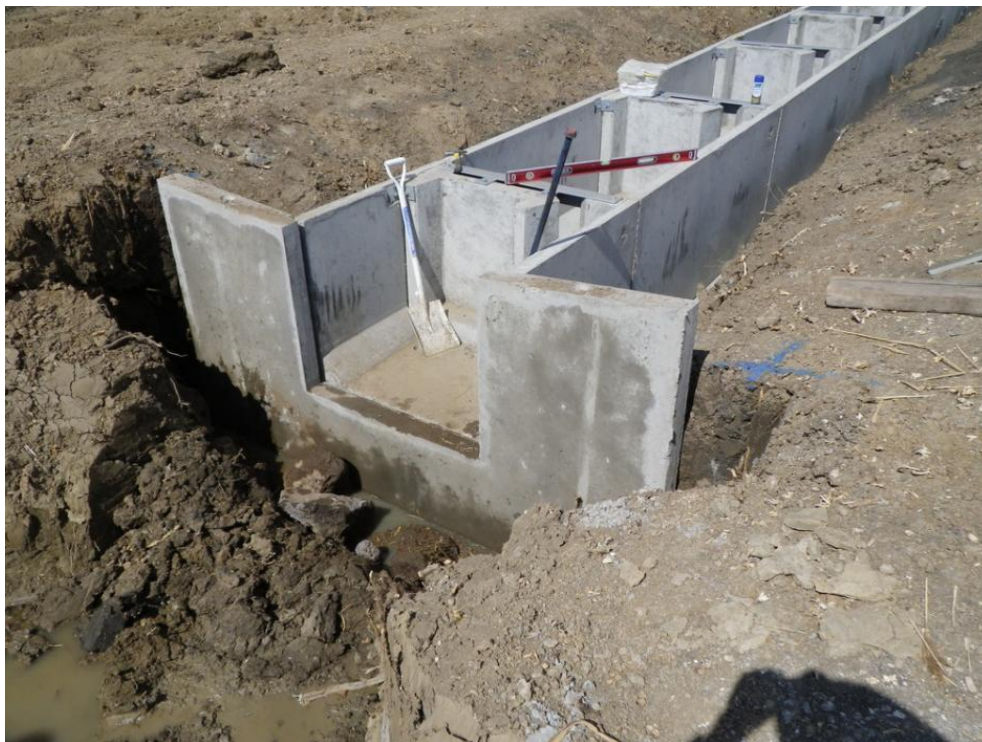
Cutoff walls were placed at upstream and downstream end of fishway.
